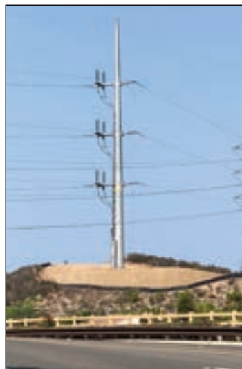
A 160-foot-tall, 230 kilovolt transition pole installed by SDG&E towers above Stonebridge Parkway near Stockwood Cove. The images demonstrate the visual impact on the parkway. (photo by Cynthia Kurose)
