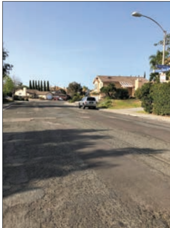
LEFT: The north end of Sunset Ridge Drive reveals significant road damage, including cracking, uneven patches and loose gravel. RIGHT: The SDG&E transmission line project, scheduled for completion in June 2018, causes delays on Pomerado Road near Spring Canyon Road. (photos by Cynthia Kurose)
