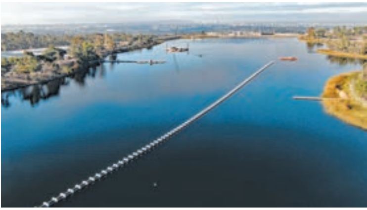
Pure Water Program pipeline at Miramar Reservoir (courtesy of City of San Diego)
