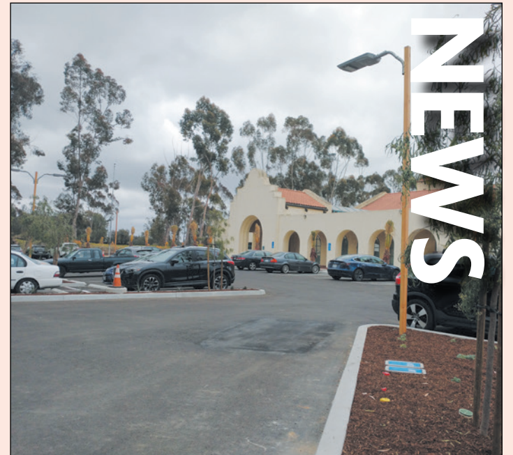
The upper lot of the Scripps Miramar Ranch Library parking lot is now open, but the lower lot is closed for expansion work. (courtesy of SRFOL)
